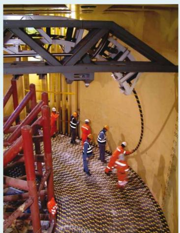
Long length of submarine cable is transported through the freighter vessel containing a static cable tank/turntable or directly loaded onto the installation vessel.
